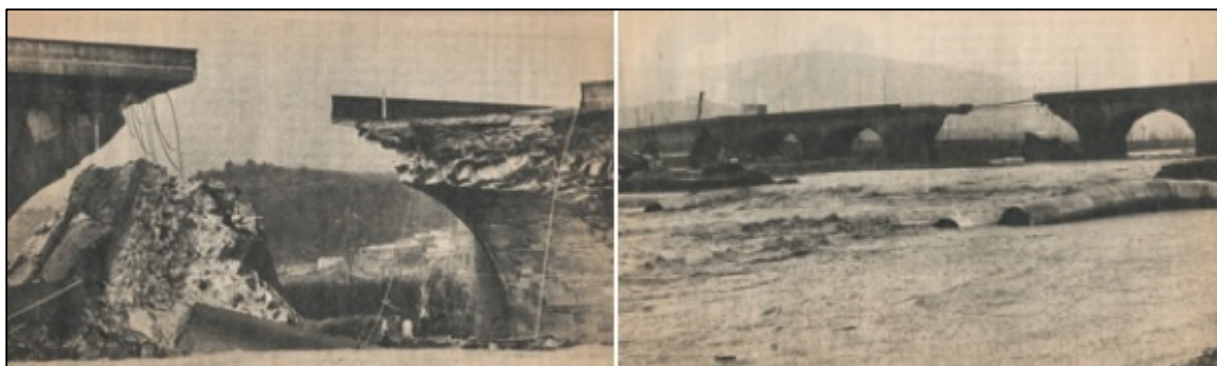
Figure 6. Images of the destruction of the bridge over the Llobregat river , at Molins de Rei (Barcelona), a few kilometres from my home, as a result of a torrential rain event in December 1971. The bridge was part of the main road between Madrid and Barcelona. These images are taken from my scrapbook, which I made in my teens, as a "weather amateur".
